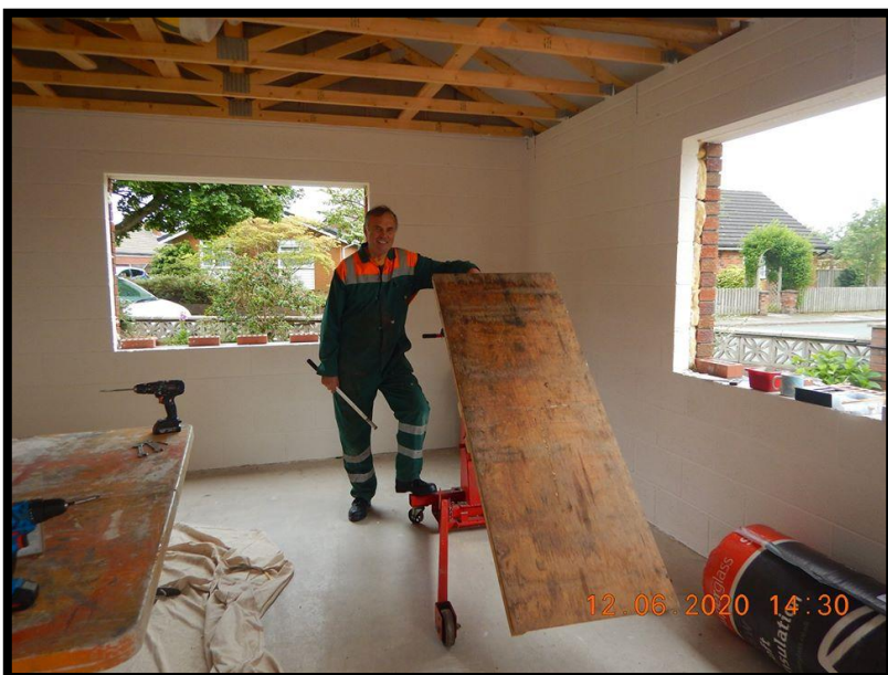
David and Tracie Baileys new garage? This has sparked much discussion on the Red Rose Facebook page – Craft room or Garage? Not to mention David's ingenious method for lifting plasterboard making good use of the engine hoist!
